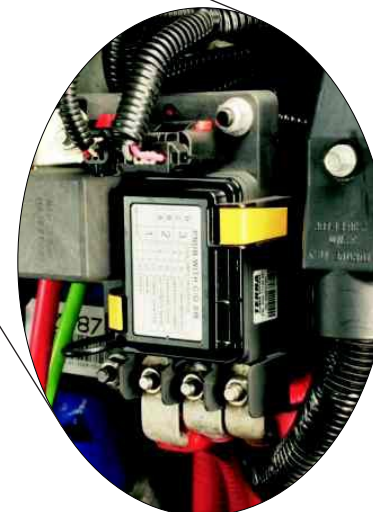
Power Net Distribution Box (PNDB) (Module 33P/281/293)
